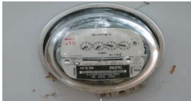
Fig. 6. A Canadian electricity meter
