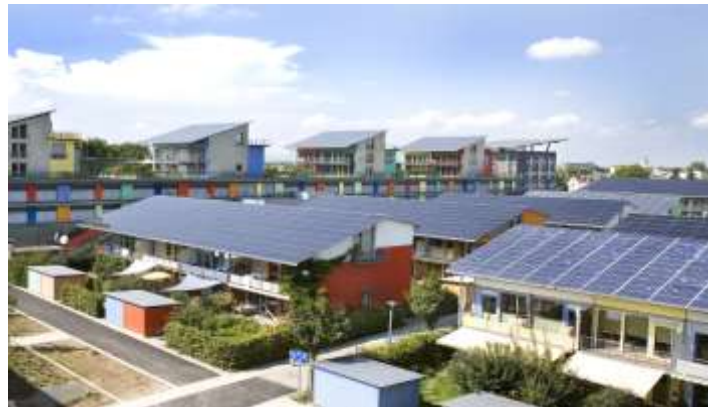
Fig 7. Rooftop solar PV systems
